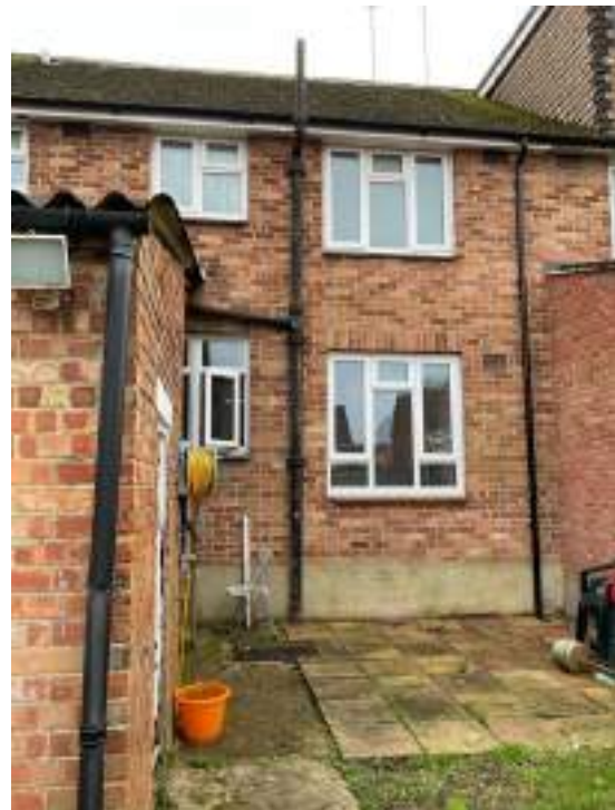
Downpipe to rear
