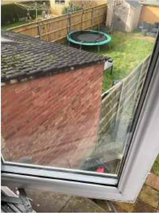
party wall agreement in place check required
