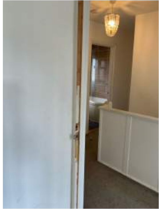
Wood work condition
