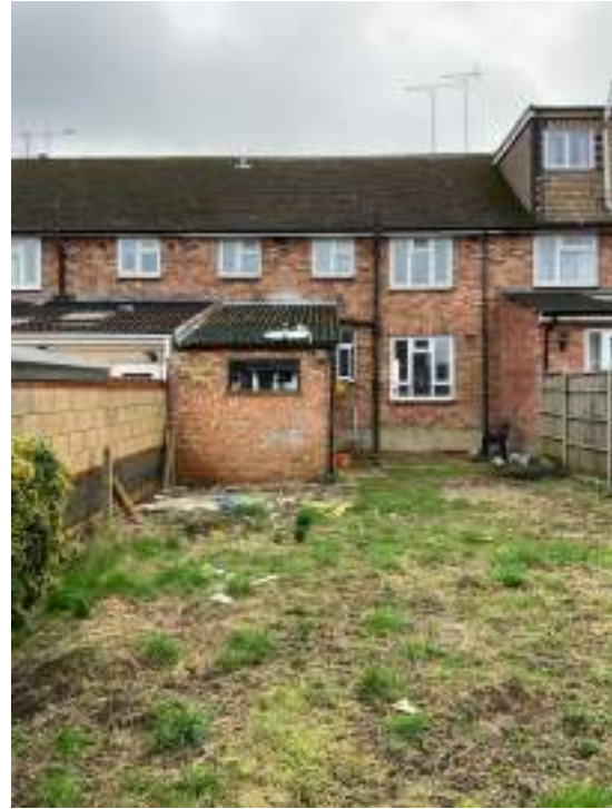
Asbestos roof to outbuilding
