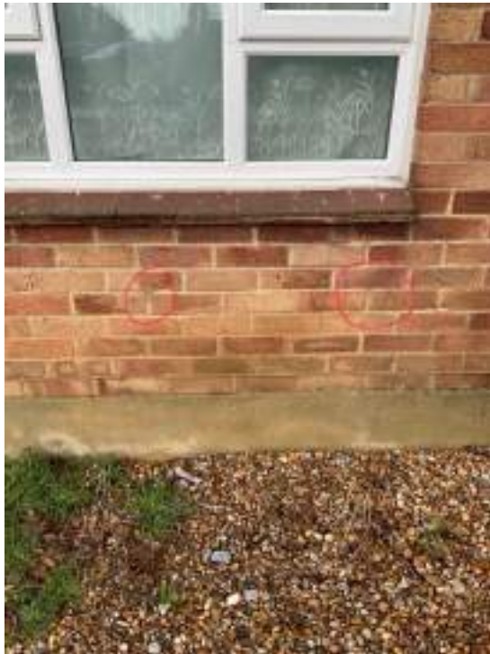
Cavity insulation holes
