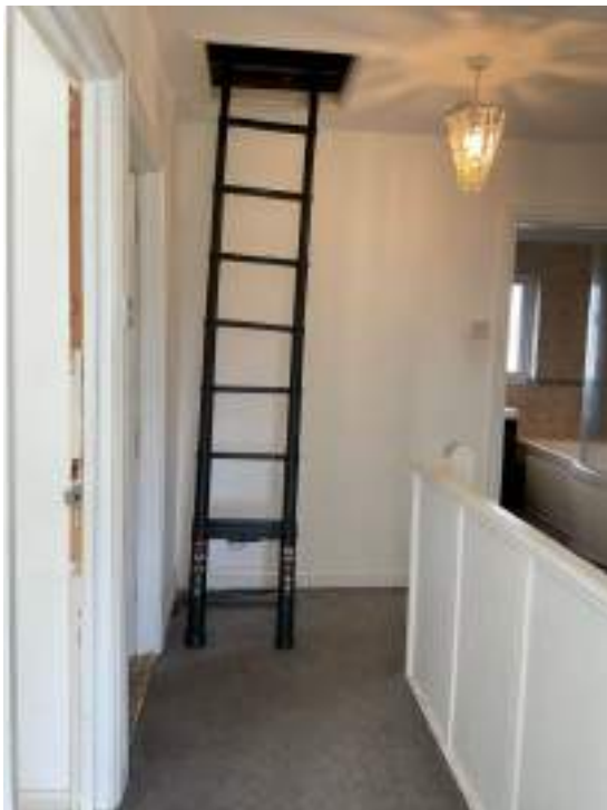
Access via hall
