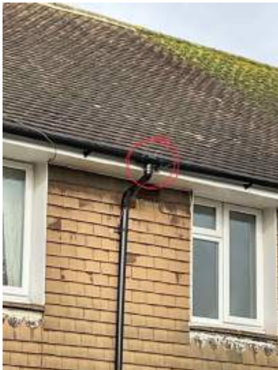
Blocked by vegetation Front elevation
