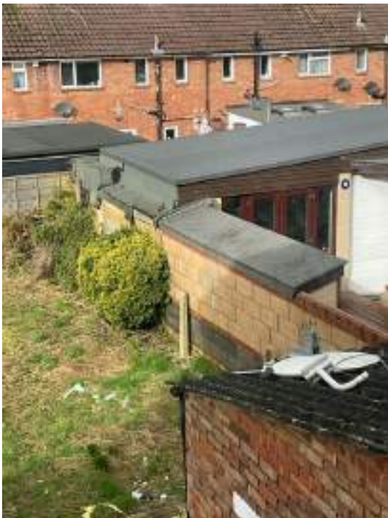
Party wall agreement in place check required
