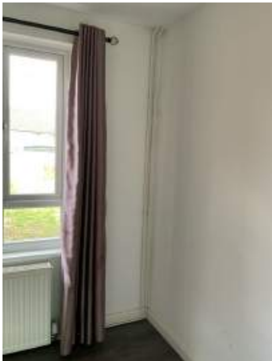
Exposed pipes can burn children and small pets
