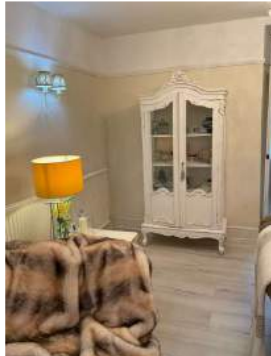
Dehumidifiers would be beneficial
