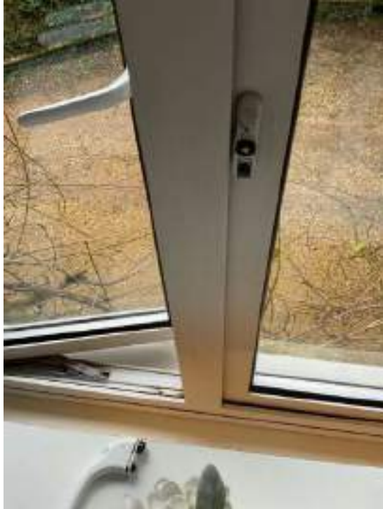
Handle broken off when testing
