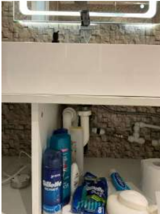
No leaks noted
