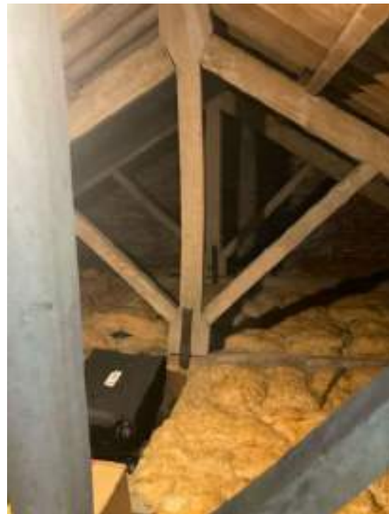
Roof with limited access to all parts
