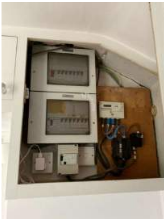
Consumer unit and meter EICR required
