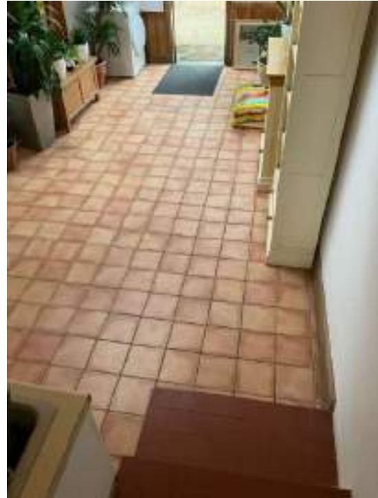
Utility floor and ground floor solid with no damp proof membrane
