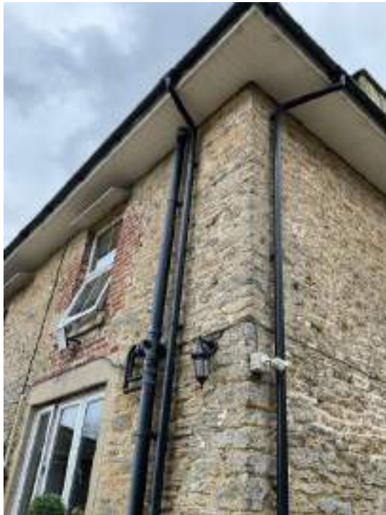
Downpipes to building
