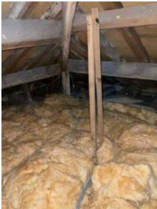
Limitations within the roof void
