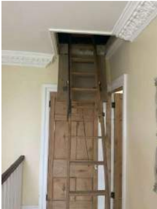
Loft access via hall hatch
