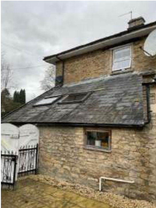
Utility roof covering
