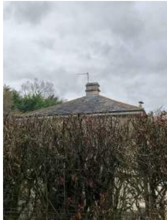
Roof and stack view and condition
