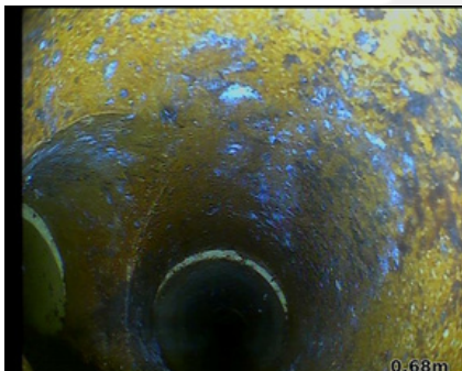
Observation [4]: Left hand lateral connection
