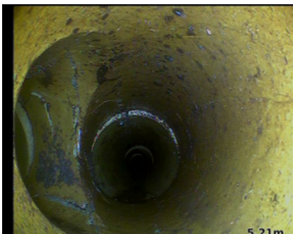
Observation [13]: Left hand lateral connection badly cracked
