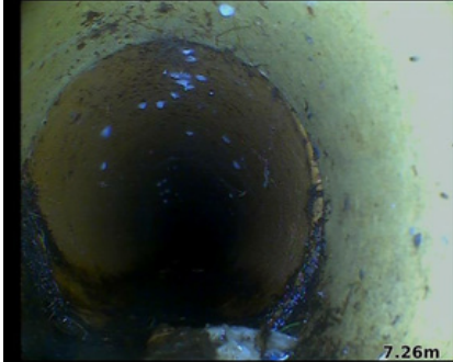
Observation [14]: Joint displacement
