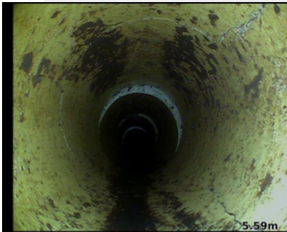
Observation [15]: large cracking
