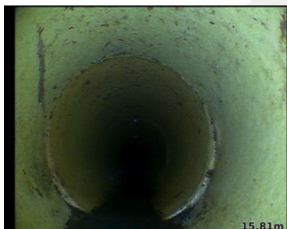
Observation [28]: Joint displacement
