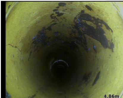
Observation [12]: Cracking from 12 o'clock
