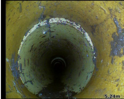
Observation [14]: Joint displacement and cracking
