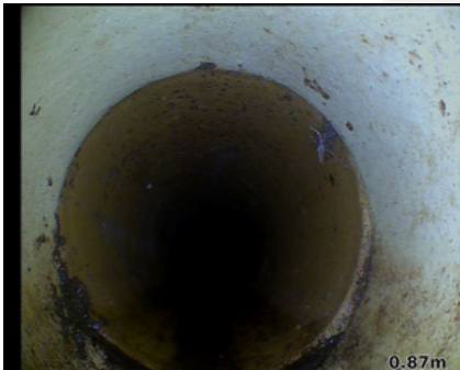
Observation [4]: Joint displacement
