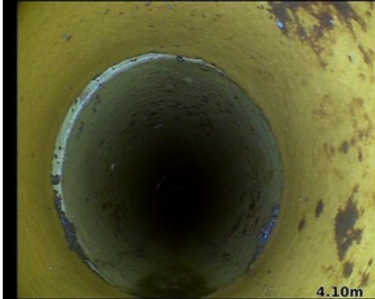
Observation [10]: Joint displacement
