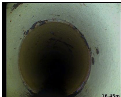
Observation [29]: Joint displacement
