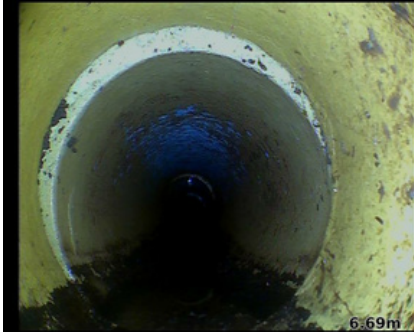
Observation [18]: Joint displacement
