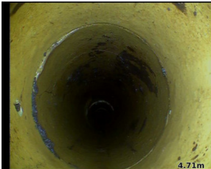
Observation [11]: Damage at 9 o'clock
