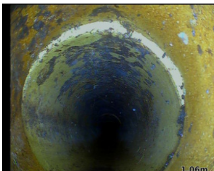
Observation [5]: Joint displacement
