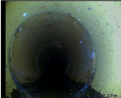
Observation [6]: Joint displacement with scale build up
