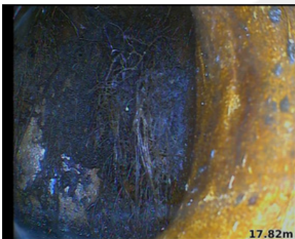
Observation [32]: Buchan trap with root ingress
