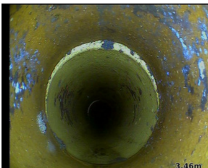
Observation [9]: Joint displacement
