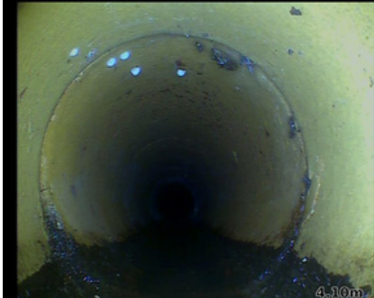
Observation [8]: Joint displacement and cracking at 3 o'clock
