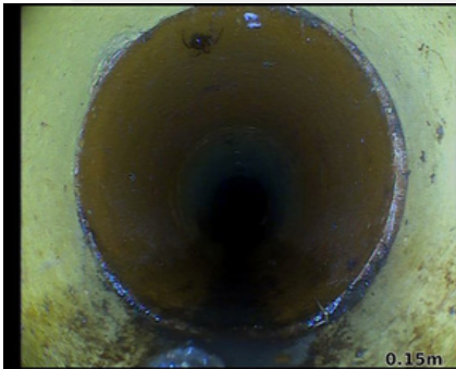
Observation [3]: Joint displacement
