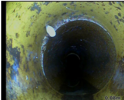
Observation [3]: Joint displacement and cracking
