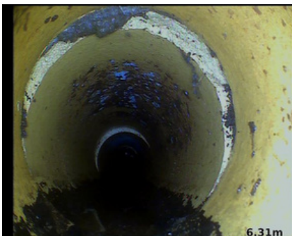
Observation [17]: Joint displacement
