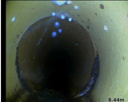
Observation [16]: Joint displacement with root ingress
