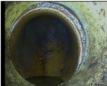
Observation [20]: Joint displacement
