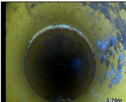
Observation [8]: Joint displacement
