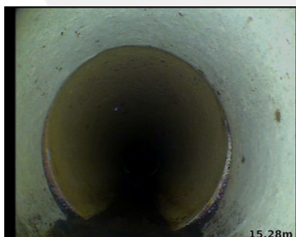
Observation [27]: Joint displacement
