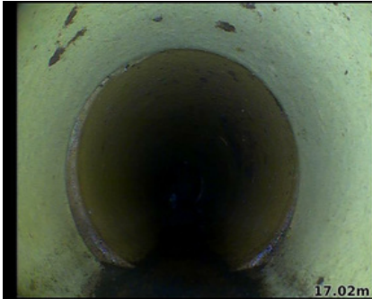
Observation [30]: Joint displacement
